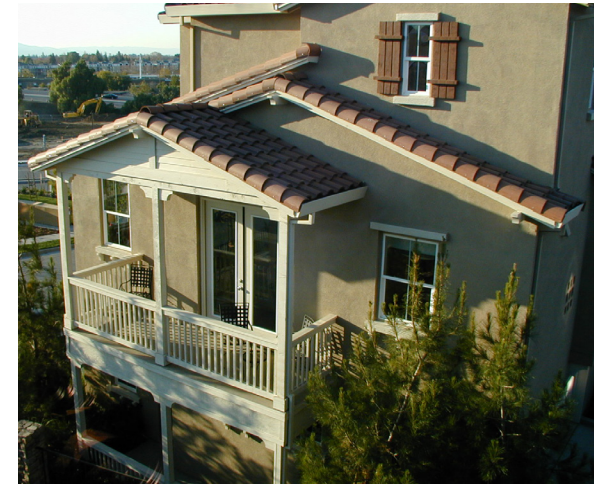
Figure 2.17.1: Balconies shall be made of wood or metal, and may be open or covered.
