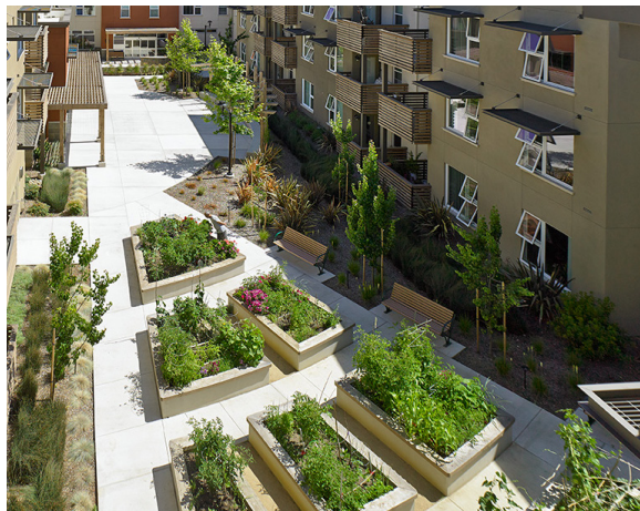
Fig. 4.8.6: Bioretention planters help manage site stormwater runoff as well as run-off from building roofs using downspouts.
